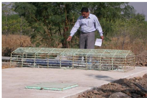
Underground water tank with filter
