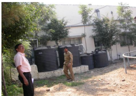
Rain water harvesting Tank near Semen bank
