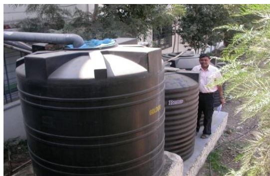
Sintex tank for rain water harvesting for semen lab
