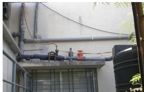
Rain water harvesting tank filter
