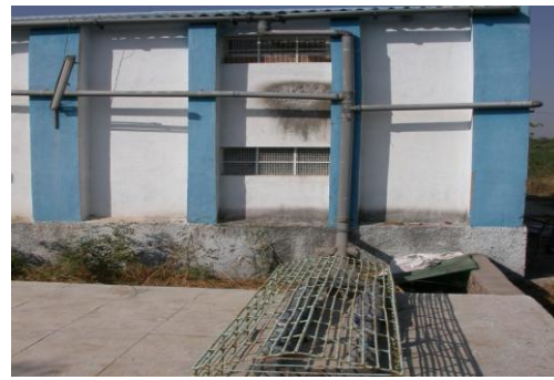
Rainwater harvesting tank & filter
