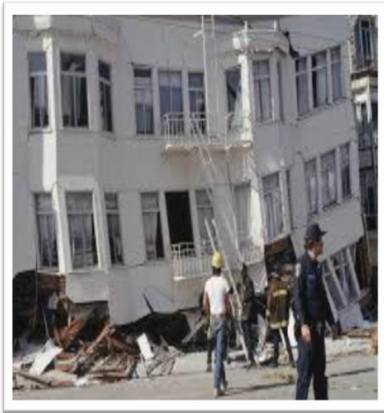
Fig.1(c): Failure of soft storey building during Earthquake in San Francisco
