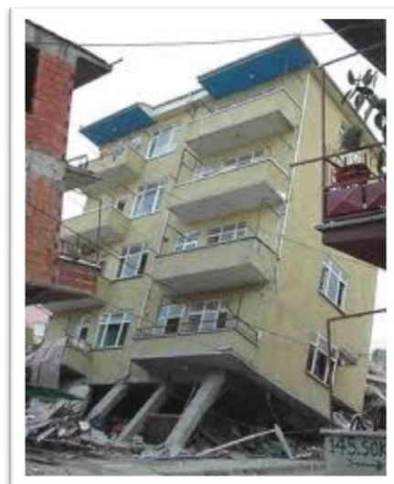
Fig.1(b): Failure of soft storey building during Earthquake in Turkey
