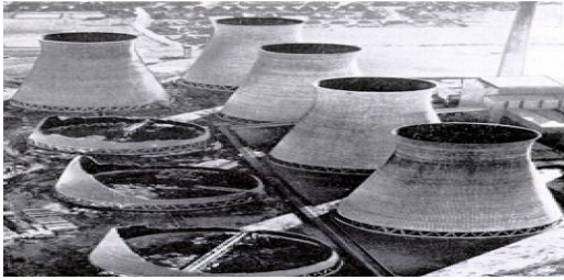
Figure 3: FerryBridge Cooling Tower Collapse
