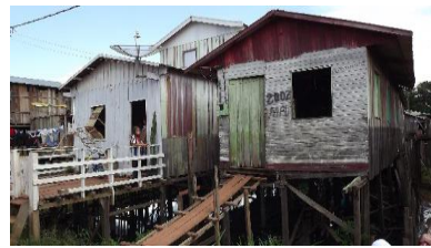
Figure 2- Buildings in risk location, in the Correnteza neighborhood. April 2016. Source: registered by Autor's
