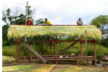
Figure 6 - Hut in construction with roof of straw, registered in the community of Canabuoca 1. April 2016. Source: registered by Ana Carolina Brugnera.
