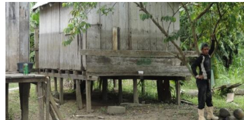
Figure 8 - shows the dislocated pillars and flooded level of water. Source: Picture by Ana Carolina Brugnera.
