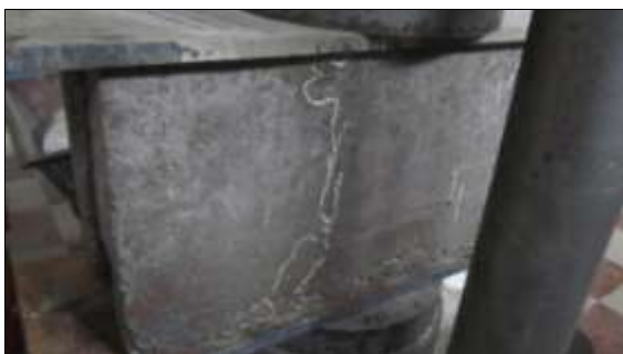
Fig 15. Failure Pattern of SHB
