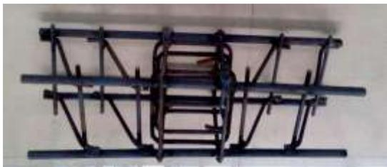
**Fig.3 Reinforcement of Beam RSBG**
