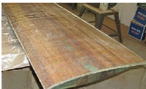
Fig: 1 Manufacture of the glass /epoxy composite beams
