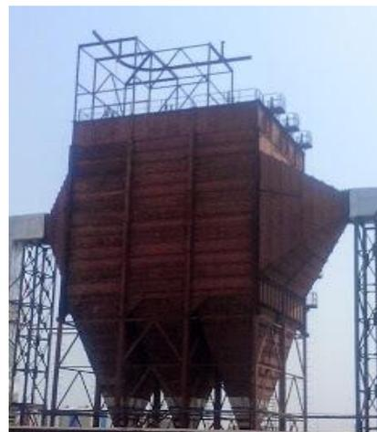
**Figure 6 - Onsite Equipment of ESP**
