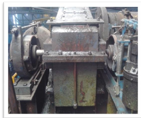
Figure 1: Shaft in the gear box of overhead crane
