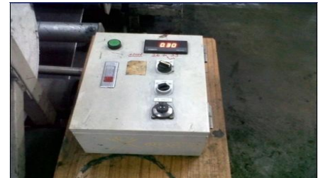
Fig. Control Panel of Drive
