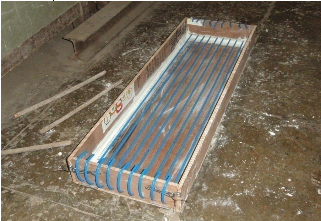
Fig. Shuttering for test specimen fitted with void formers
