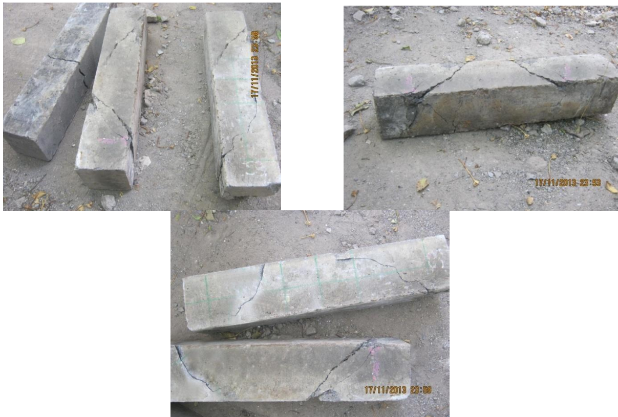
Fig. 3 - Typical crack patterns ( a/d = 2 ).
