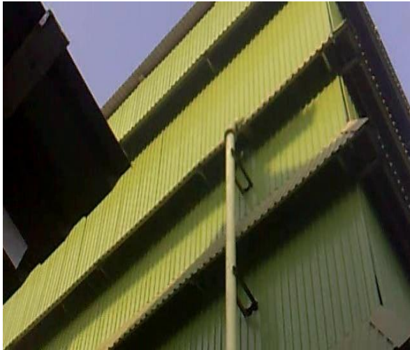
Fig.3.Before implementing M.S. bend pipe having inside cast basalt coating
