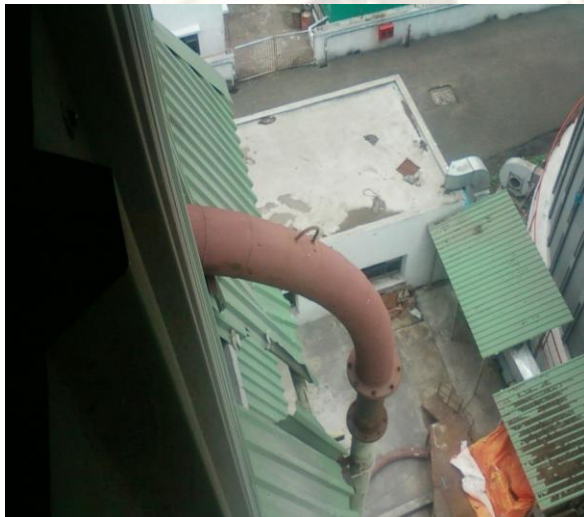
Fig.4.After implementing M.S. bend pipe having inside cast cast basalt coating
