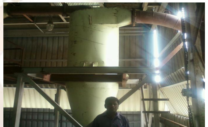
Fig.7A. After implementing cyclone separator in between bag filter and blower (With bend pipe and cyclone separator)
