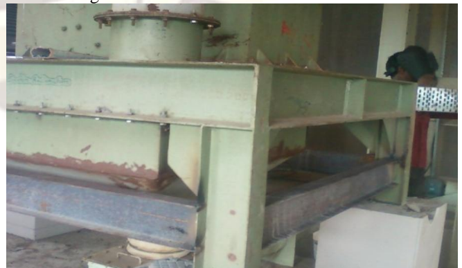
Fig.10. Hammer mill after connecting 'I' beams between the Supports
