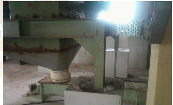
Fig.9. Hammer mill after vibration and breakage of concrete base
