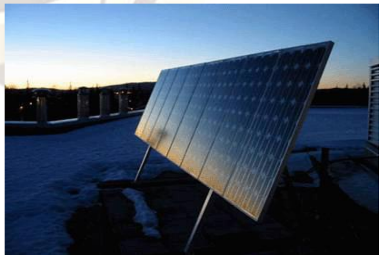
Fig-2 Photovoltaic (solar) panels
