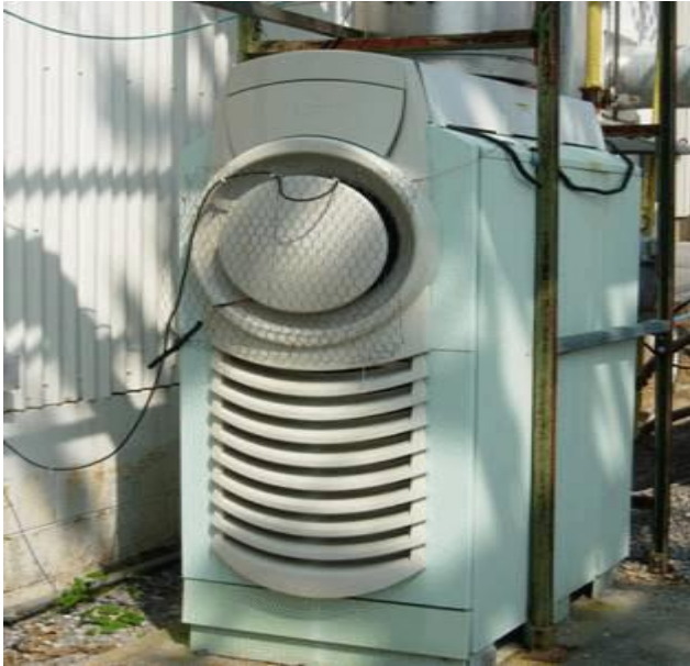
Fig-3 A 300KW Micro-turbine at Oak Ridge National Laboratory, TN
