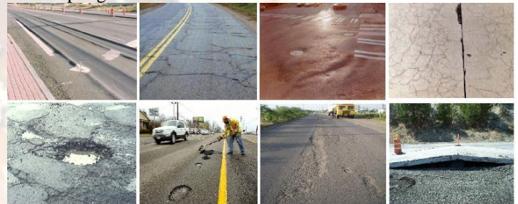
Photograph 1 Different Types of Distress on Highway Pavement
