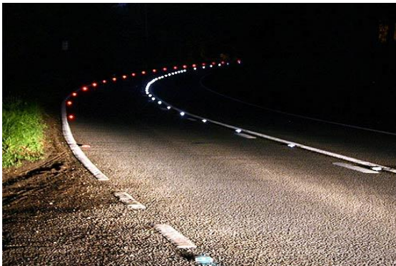
Fig: 3 Illuminated Highway at Night
