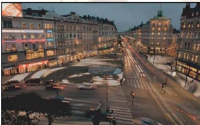
Image 4.2 showing the illuminated road incorporated with translucent concrete underneath it.
