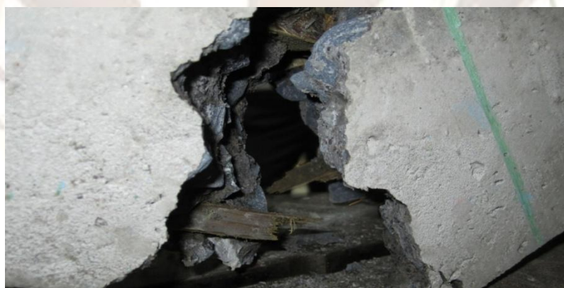
Fig.17: Failure of Doubly Reinforced Beam
