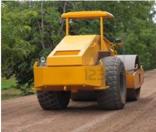
Figure 1.0: Field Compaction of the Test Area.
