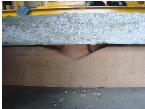
Fig. 15. The holes of the concrete slab aligned accordingly along the timber notches with the shear connectors still visible to sight from the side view
