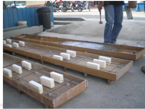
Fig. 12. Polystyrene blocks as the mould to form connection pockets on the concrete slabs
