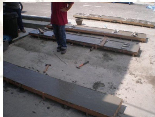
Fig. 13. Concrete slabs left to cure for 28 days from the day of concrete casting session with the polystyrene blocks resting in place
