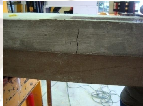
Fig. 25. Crack spotted on the concrete topping close to the support
