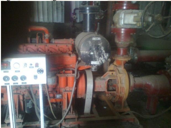
Fig.6 Engine control panel.
