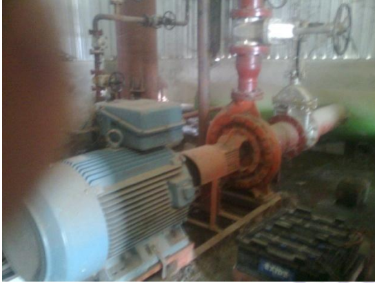
Fig.4 Main fire pump.
