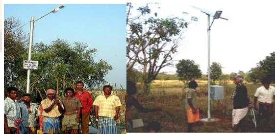
Fig.8 : Village street light
