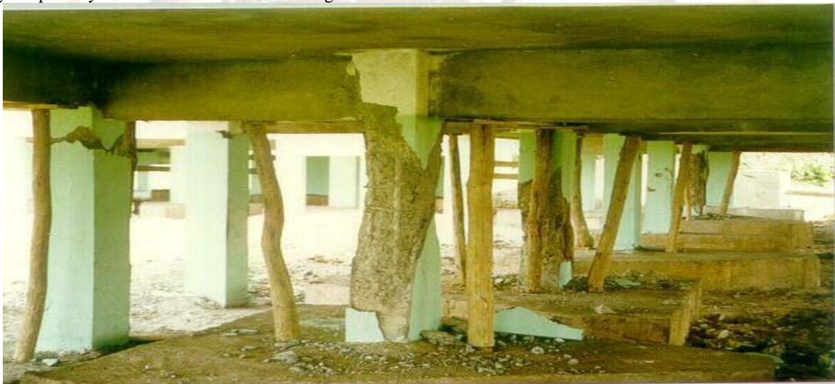
Figure 2 :: Damage to columns in the stilt storey of Youth Hostel building.
