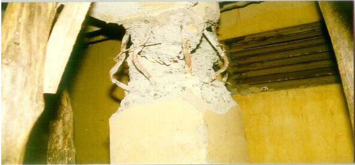
Figure 1 :: Damage to columns in Hingiri apartment.
