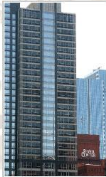
Fig. 4: Sky scrapper Building with irregularity
