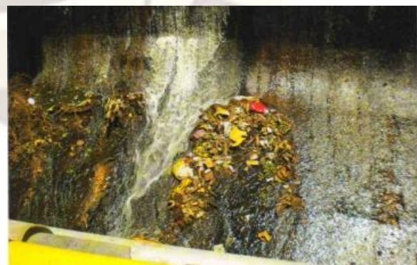
FIGURE.2 GARBAGE DEPOSITED BENEATH THE SPILLWAY
