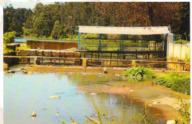
FIGURE.3 SCREENING AT ENTRY POINT
